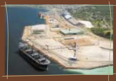
Loading of woodchips from the Albany port.
